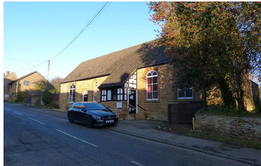
Figure 32 Newnham Village Hall, Church Street.
